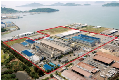
The world's largest isotropic graphite plant, Takuma Division
