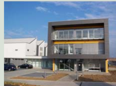
The new factory at Toyo Tanso's German subsidiary
